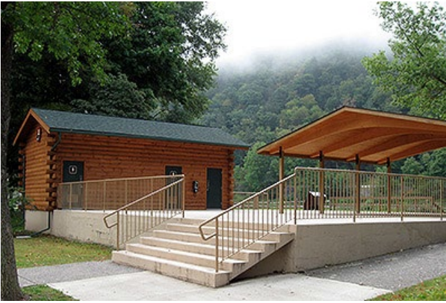
Bathroom facilities at Kittatinny Point Visitors Center
